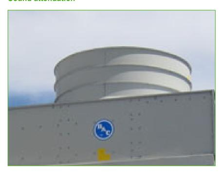
PFI cooling towers use **quiet and low kW axial fans**, but to reduce noise even further, you can extend your PFI cooling tower with <u>sound attenuation</u>:
