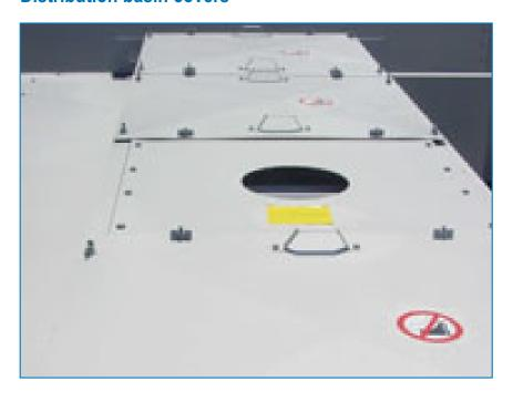
Distribution basin covers on units prevent contamination of basin water due to debris etc.
