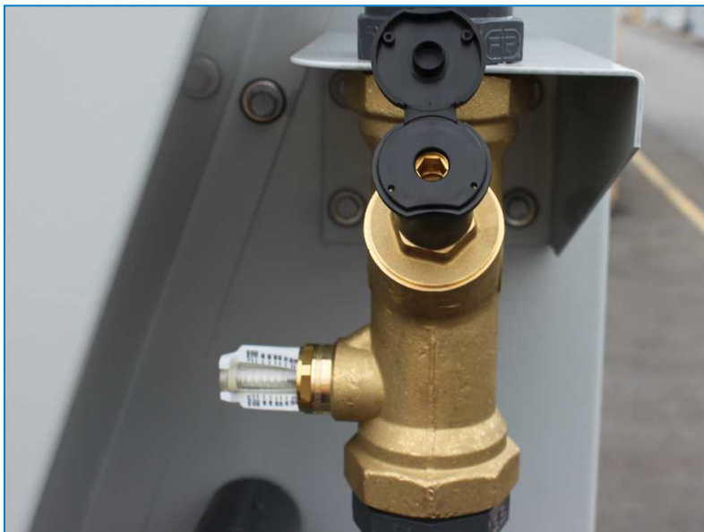
Water flow adjustment screw
